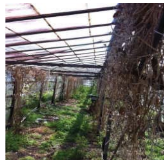
View of: Glass house Inspected on 18.09.2013
